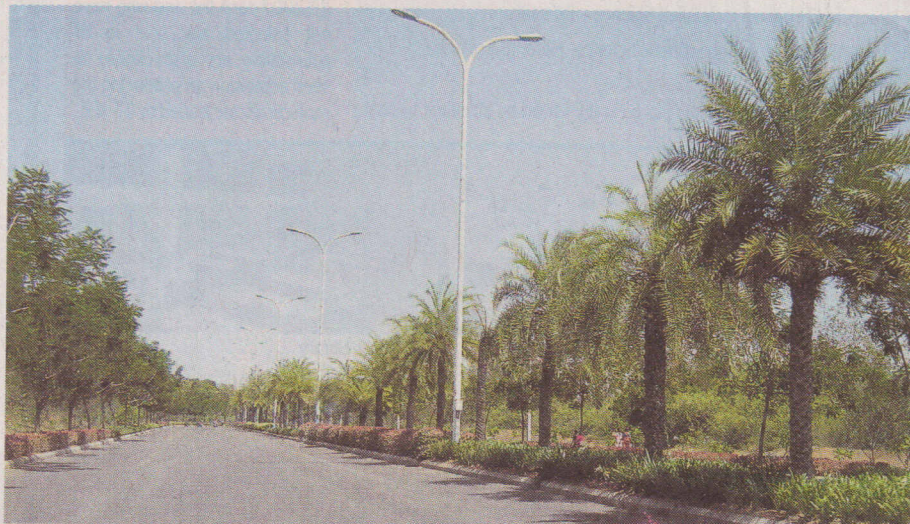
A NEW ERA: Six-lane road at Mahindra World City near Chennai.
